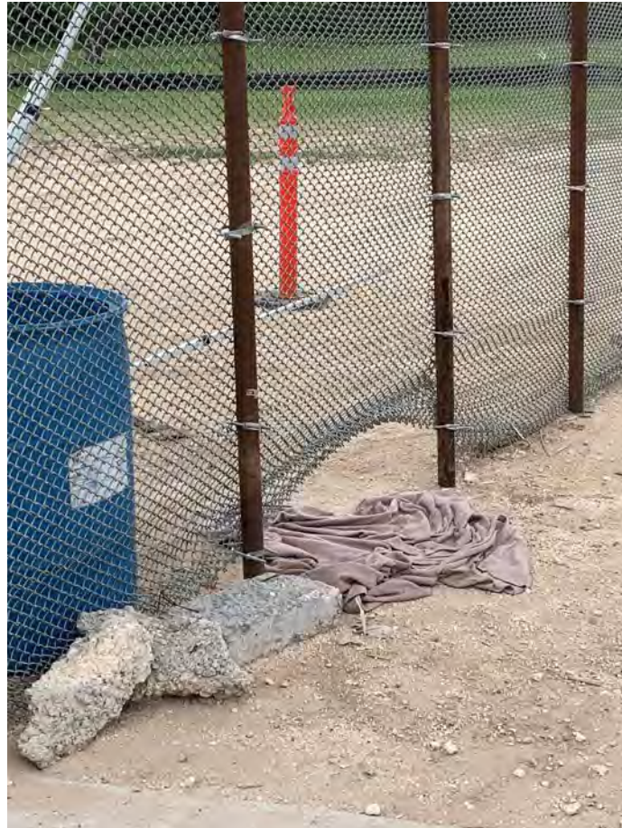
Figure 3: Evidence of an illegal crossing beside the unfinished “border wall”
